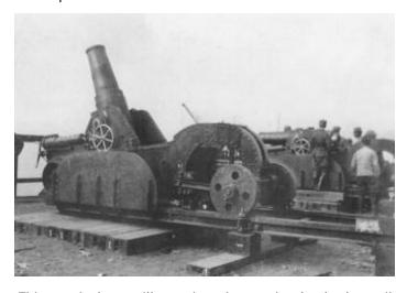
This particular artillery piece has a simple dual recoil operating mechanism: a hydraulically controlled reduction of the gun cheeks that hold the trunnions, and a hydraulically reduced carriage in track that carries the gun cheeks. Both return to battery on inclines by gravity. For movement, the gun was removed from the emplacement and transported on its wheels. The emplacement components are moved separately.
